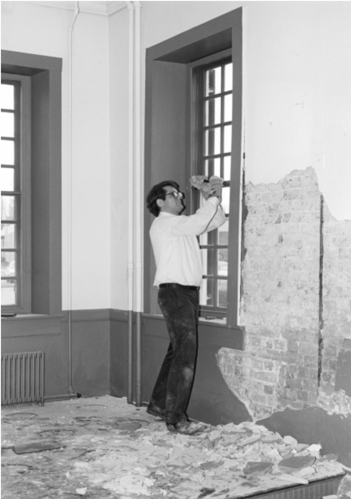
An architectural historian exposes brickwork to study eighteenth-century construction features.
